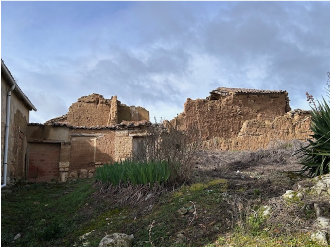
Illus.2 Remains of the former Cabezón residence
